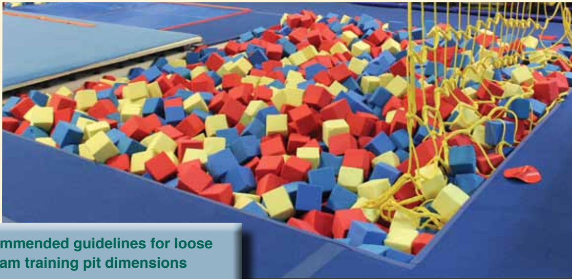
This foam pit was six feet short of recommended guidelines, causing our client to strike his head on the pit's rear ledge and resulting in partial paralysis.
